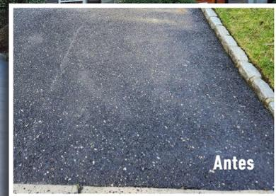
Powder pigment was added to the Surface Armor™ to achieve a similar finish to the original asphalt. The 1250 ft<sup>2</sup> driveway was completely resurfaced in approximately 5 hours.
