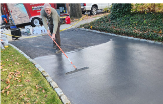
Driveway is given a new visual and service life with a final application of Ecobeton-USA® Vetrofluid®.
