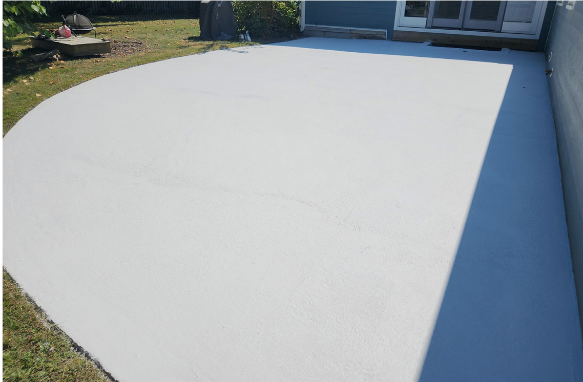
The patio brought back to 'new' appearance and ready for use.
