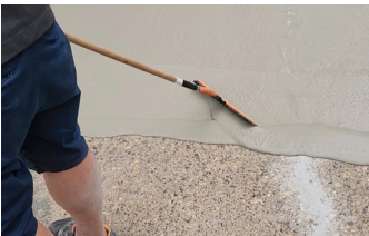
Two coats of Surface Armor™ are applied with a GST Squeegee Trowel.
