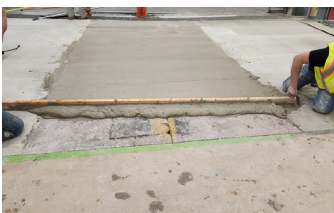
The center panel is filled with Elephant Armor® to the level of the two outside panels.
