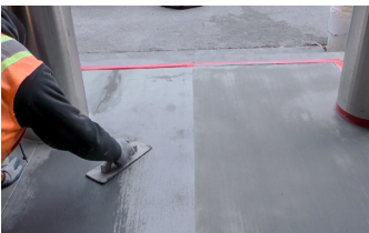
Using a trowel to complete first coat of Surface Armor®.
