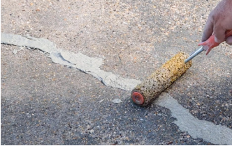
Elephant Armor® is used to fill deep cracks.
