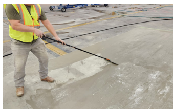
A coat of Surface Armor® is applied over the entire repaired (filled) area.
