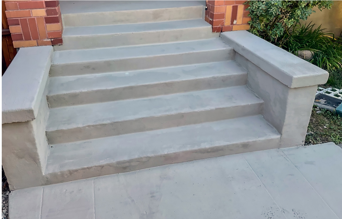
Restoration complete in 5 hours using one bag of Elephant Armor® DOT and one bag of Surface Armor™ without the need for the traditional and extremely costly, time consuming deconstruction/reconstruction process greatly extending its life-cycle.
