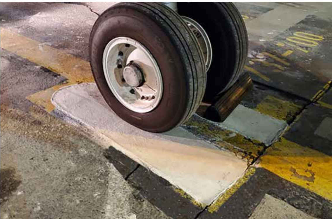
Damaged concrete surface unsafe for use.
