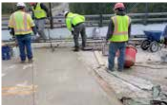
Putting final finish on new bridge link.
