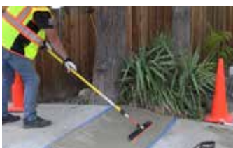
Preparing the surface for a broom finish.
