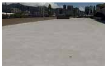
Repair complete and ready for use.
