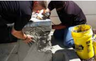
Applying Elephant Armor® - DOT to the vertical surface without forming.
