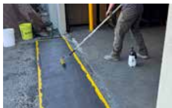
Using GST Texture Roller for final placement.
