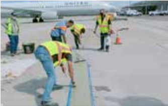
Elephant Armor® cap is placed using an edging trowel and squeegee.
