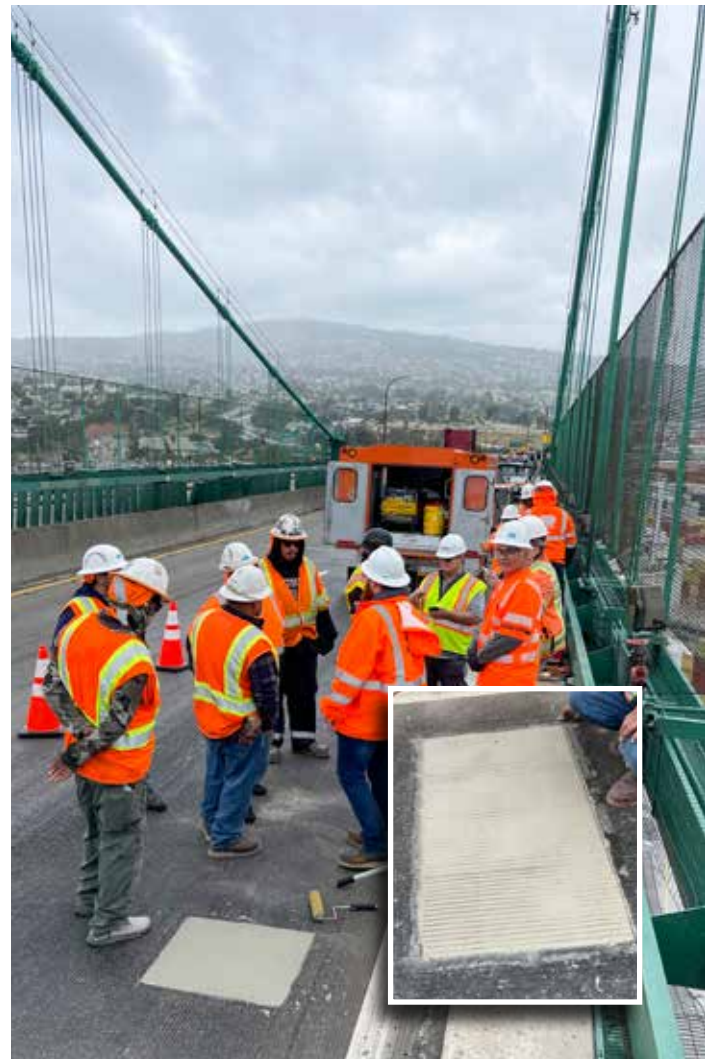
Elephant Armor - DOT ease of use and quick set time, allowed the pothole to be permanently repaired with a minimum disruption to traffic. This lane was back to service in less than 3 hours!
