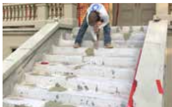
Filling larger cracks prior to full encapsulation.
