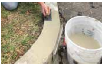
Finishing curb repair with edging tool.
