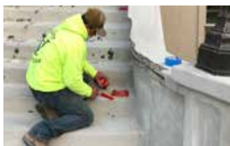
Severely broken and degraded wall cap.
