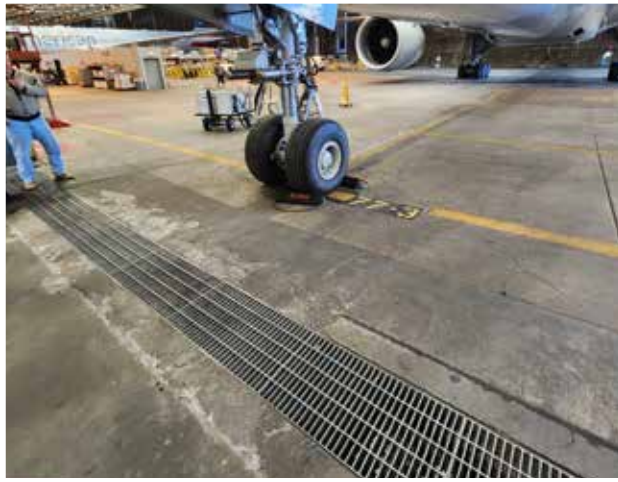
Photo showing extensive damage to the concrete around the drains, including a 3" 'point load' depression in the parking area at the jet's nose gear.
