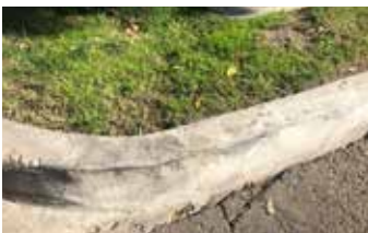
Finished curb can take immediate vehicular abuse.
