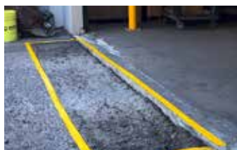
Rehabilitation of warehouse ramp transition reducing costly forklift maintenance.
