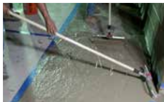
Applying second lift of Elephant Armor®.
