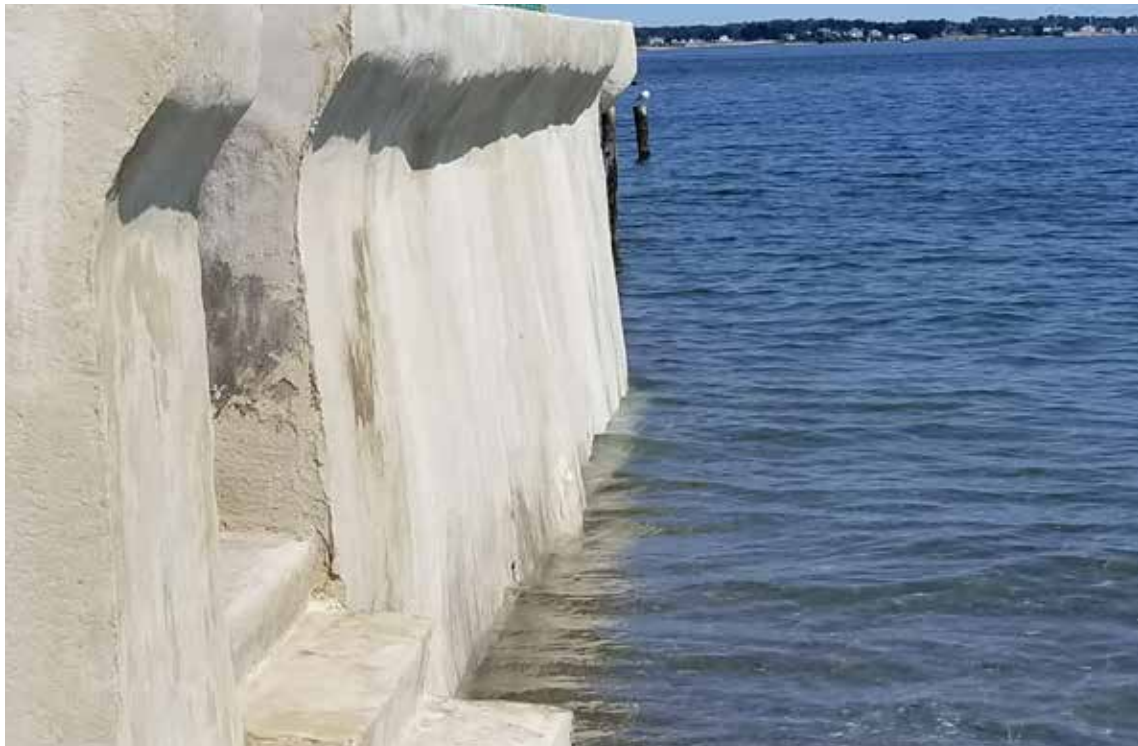
Full degraded seawall encapsulation completed between tides.
