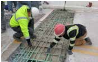
Elephant Armor - DOT's flowable mix ensures steel encapsulation.
