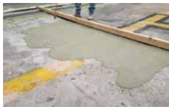
Elephant Armor®-DOT is applied in 3 panels to fill and level the repair area.
