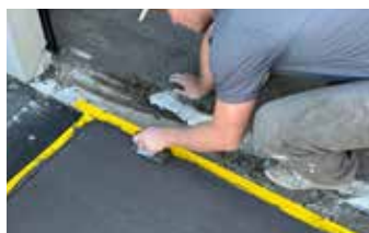
Finishing edges with an edging trowel.
