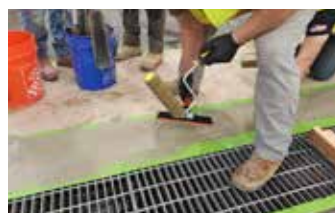
The second damaged area on the outside perimeter of drain is now overlaid with Elephant Armor®-DOT.
