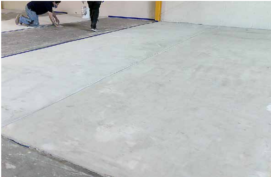
The installation was completed using Elephant Armor® - DOT in sections allowing for uninterrupted use of the warehouse, saving 80% of the original remove and replace estimate.
