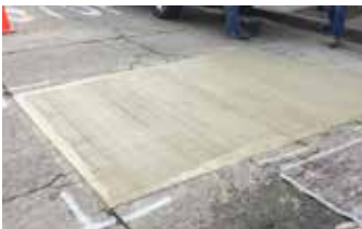
Repair completed in two hours and open to traffic in four hours.
