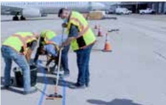
Filling cracks with Elephant Armor® using a roller and squeegee.
