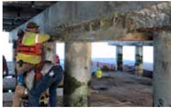
Placing Elephant Armor® over the properly primed surface.
