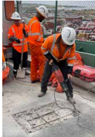
The damaged surface is removed and any loose material is cleaned away with a broom and a blower.
