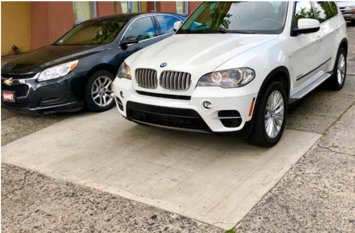
Repaired road panel 7 years after installation is still performing perfectly. With minimal environmental impact by significantly reducing the time of repair, a new lifecycle is achieved while also reducing repair costs by as much as 50%.
