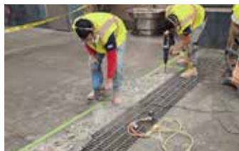
All loose unstable concrete is chipped away to provide a solid surface.
