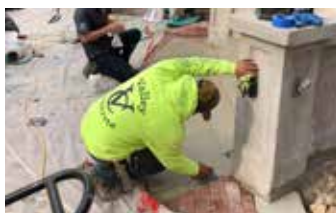
Finishing vertical wall repair.
