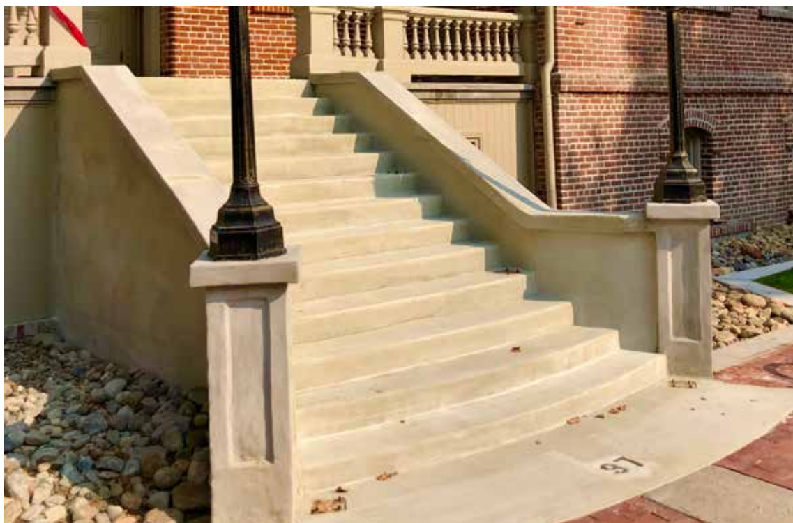
Damaged concrete stairs overlaid without deconstruction or forming, saving time, money and reducing the disruption of service.
