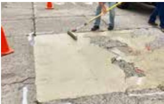
Application of quarter inch Elephant Armor® - DOT overlay.
