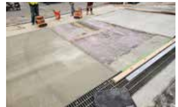
The last panel is ready to be filled and levelled with the two outside panels.
