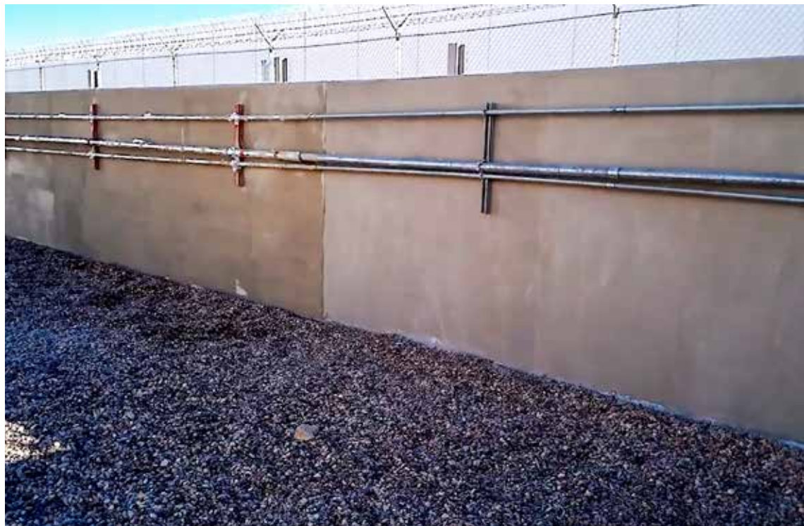
A newly resurfaced CMU block wall with a 'like new' appearance, eliminating the visual cracks and discoloration. The wall is now waterproof and structurally sound.
