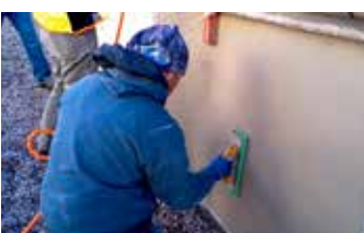
Using a grout float to apply the desired finish prior to the final application of Vetrofluid®.
