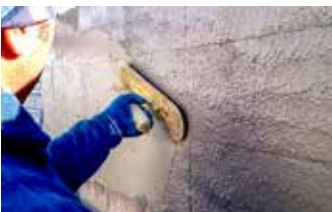
A standard pool trowel is used to spread the Surface Armor™ and achieve an even thickness.
