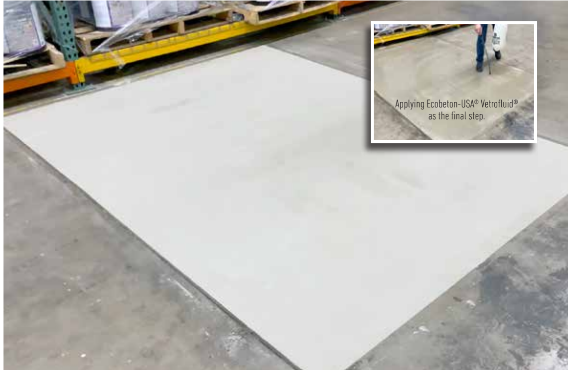
Warehouse floor panel brought back to 'new' appearance and ready for heavy forklift traffic. A light broom finish was applied to reduce a 'slip and fall' hazard.
