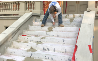
Filling larger cracks prior to full encapsulation.
