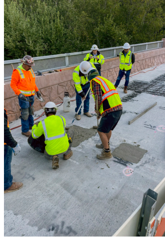
Applying Elephant Armor® - DOT as a fill material around the exposed steel.
