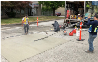
Finishing placement of quarter inch Elephant Armor® overlay.
