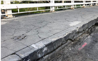
Badly cracked and spalled concrete sidewalk.
