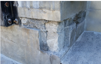
Extreme damage to loading dock.
