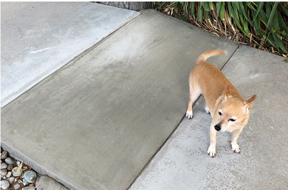
Trip and fall hazard was eliminated without having to remove the failing panel.
