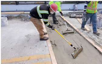
Placement of Elephant Armor - DOT using GST Texture Rollers.
