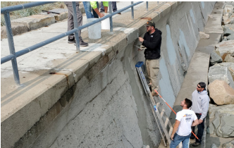
Applying Elephant Armor® to repair area.
