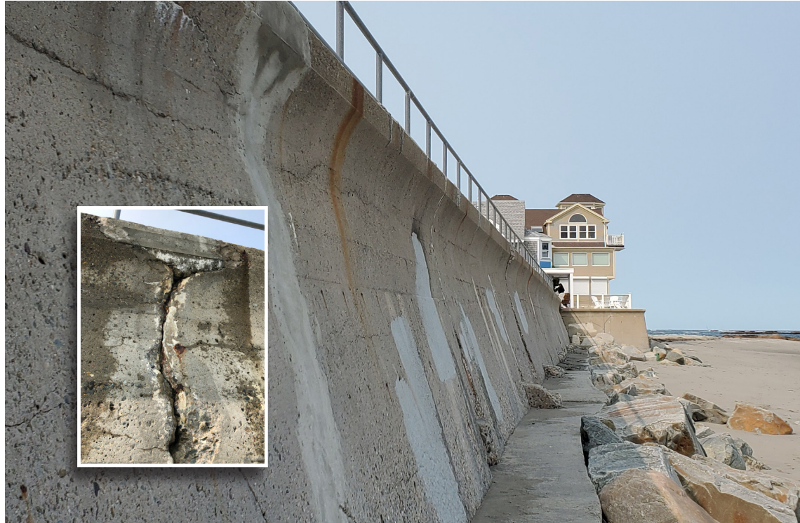
Severe fracturing of old seawall due to saltwater and weather exposure given new life using Elephant Armor® - DOT.
