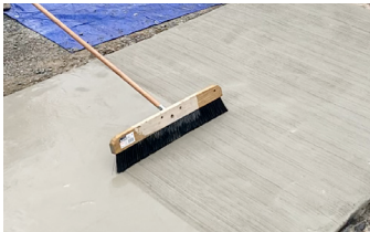
After GST Squeegee Trowel is used to smooth the surface, a broom finish is applied.
