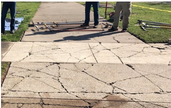
Severely cracked sidewalk panels prior to Elephant Armor® repair.
