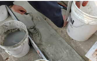
Elephant Armor® applied without using forms.
