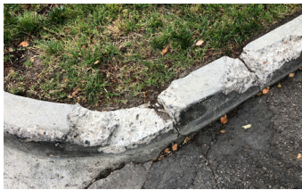
Severely damaged curb.
