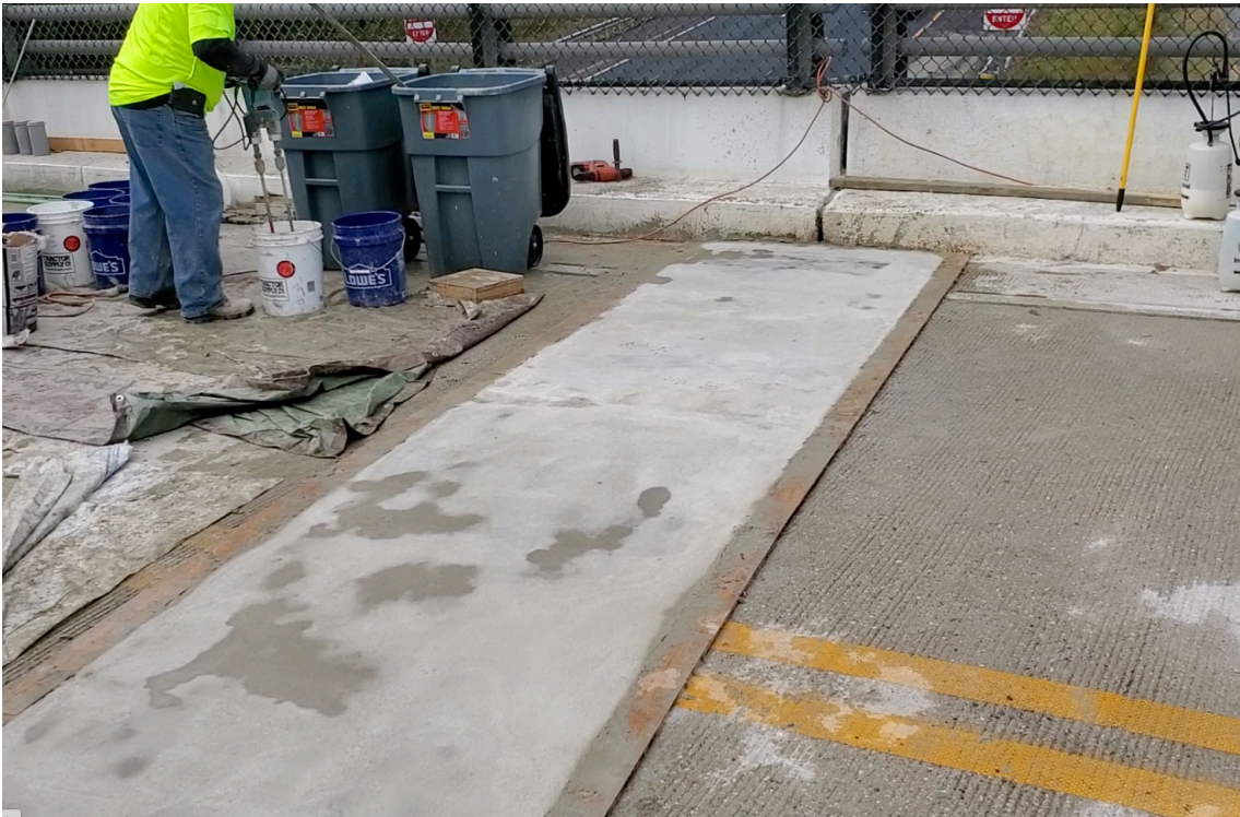
Bridge link construction completed in just 4 hours. Elephant Armor® - DOT was chosen due to its high compressive, flexural and tensile strength. Its fast setting properties allow for minimal down time and a quick return to service.
