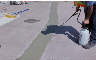
Finishing Elephant Armor® Mortar repair with an application of Ecobeton® Vetrofluid®.
