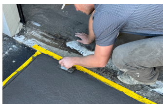
Finishing edges with an edging trowel.
