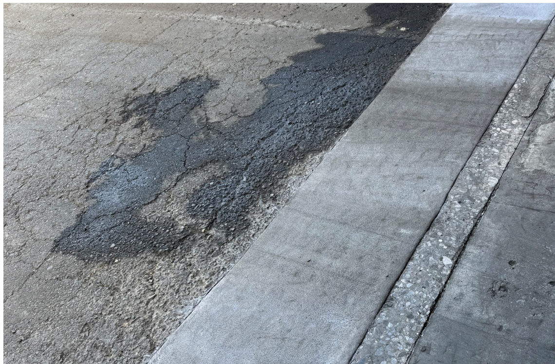
Finished ramp transition completed and ready for use in two hours.
