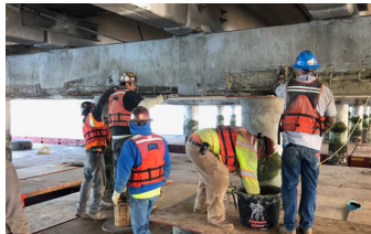
Applying a slurry primer coat over the repair area ahead of Elephant Armor® placement.
