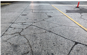
Distressed concrete roadway.
