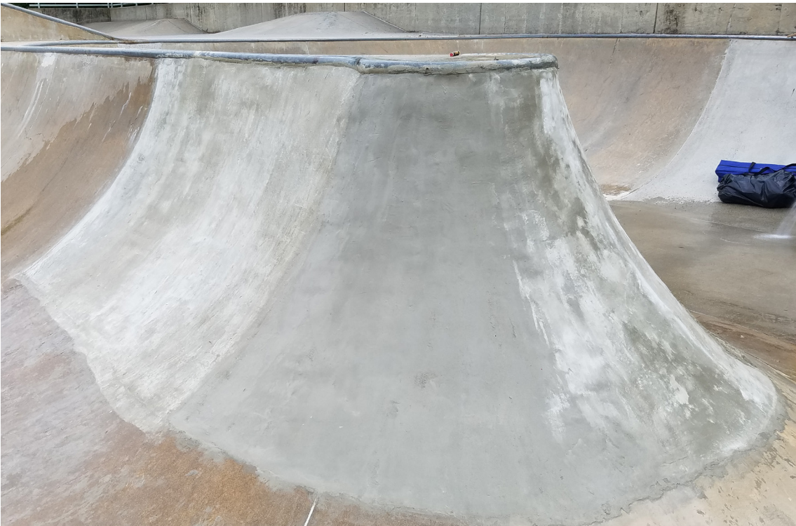
Overlay of degraded failing concrete completed with Elephant Armor® - DOT.
