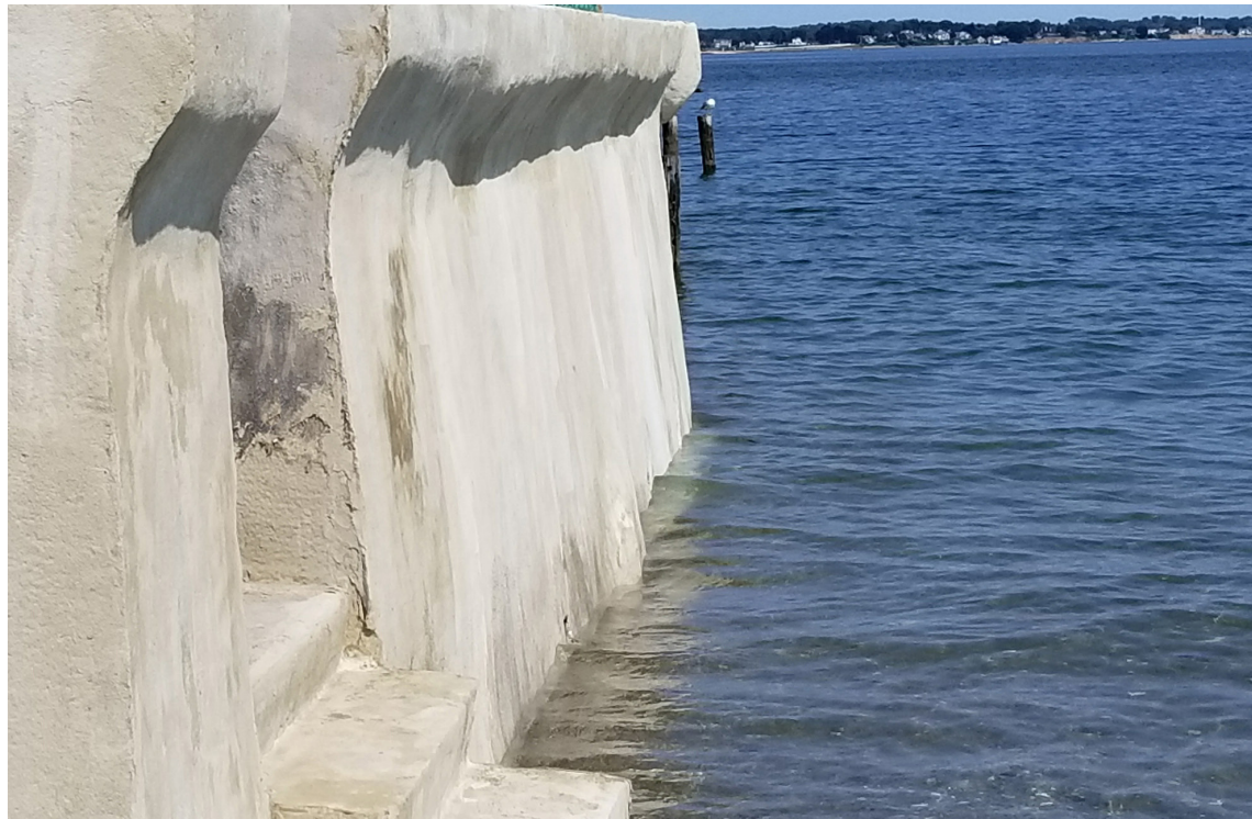
Full degraded seawall encapsulation completed between tides.
