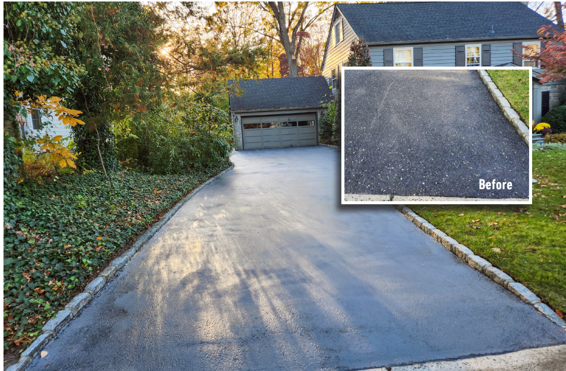
Powder pigment was added to the Surface Armor™ to achieve a similar finish to the original asphalt. The 1250 ft² driveway was completely resurfaced in approximately 5 hours.
