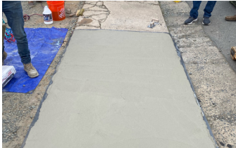
After cracks are prefilled, a 1/4" lift of Elephant Armor® - DOT is applied to the surface.
