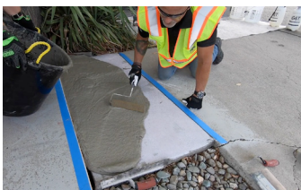
Applying Elephant Armor® - DOT using a GST Texture Roller.
