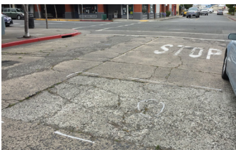
Failing road panel.
