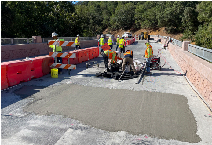
Areas with exposed rebar are filled and encapsulated with Elephant Armor® - DOT prior to final overlay application of Elephant Armor® - DOT.
