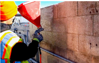
Surface Armor™ is sprayed on the degraded block wall after an initial application of Vetrofluid®.
