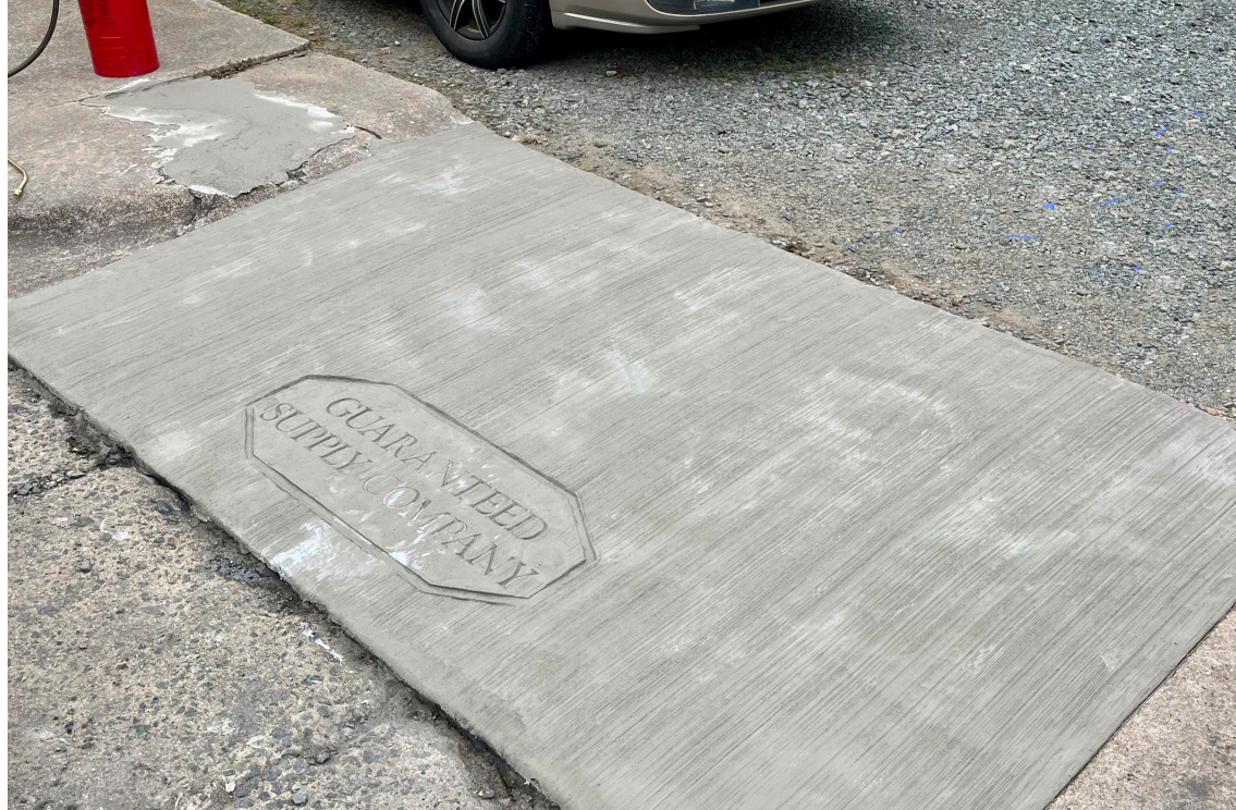
Finished repair stamped with Guaranteed Supply Company logo. Ecobeton®-USA VetroFluid® is applied as a last step after the Elephant Armor® Mortar repair has achieved a full cure.
