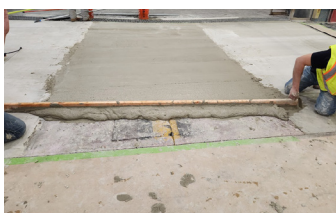
The center panel is filled with Elephant Armor®-DOT to the level of the two outside panels.
