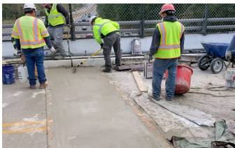
Putting final finish on new bridge link.
