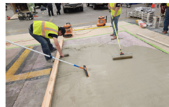
Elephant Armor® is easily placed and levelled with GST Rollers and Squeegee Trowels.
