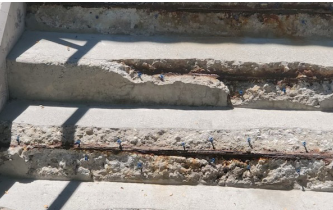
Concrete stairs degraded down to exposed steel.
