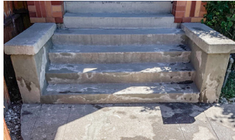
Elephant Armor® - DOT reconstruction complete, now ready for Surface Armor™ permanent micro-topping.
