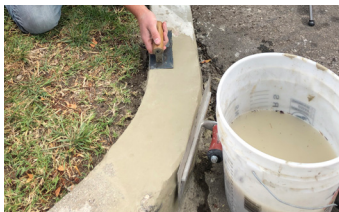
Finishing curb repair with edging tool.
