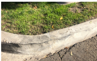
Finished curb can take immediate vehicular abuse.
