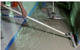
Applying second lift of Elephant Armor®.
