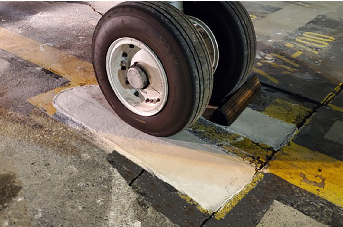
Damaged concrete surface unsafe for use.
