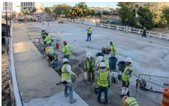
Placing Elephant Armor® using GST specialized tools.
