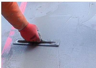
A trowel can be used to match existing surfaces.
