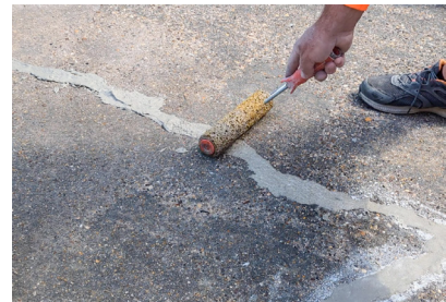
Push and flatten the DOT Mortar into cracks with a roller.
