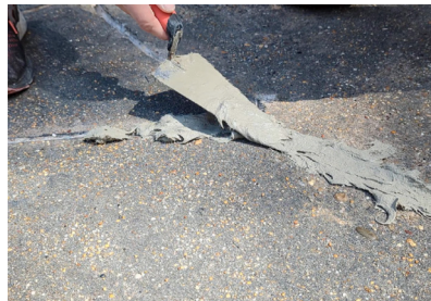
Fill cracks with Elephant Armor® DOT Mortar using a trowel.
