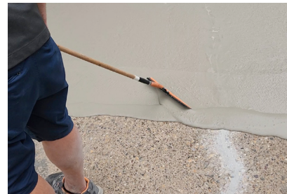
Apply a 1/32" - 1/16" (1-2 mm) coat of Surface Armor™ to the substrate followed by a second coat after curing.
