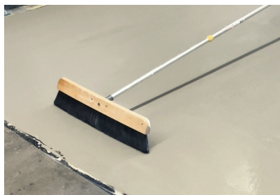
A broom finish provides a non-slip surface.
