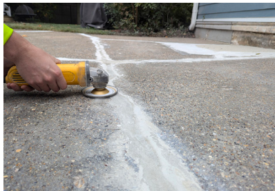
Grind the filled cracks to remove any feathered edge.
