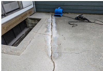
Remove any loose material from the cracks with an angle grinder and leaf blower.
