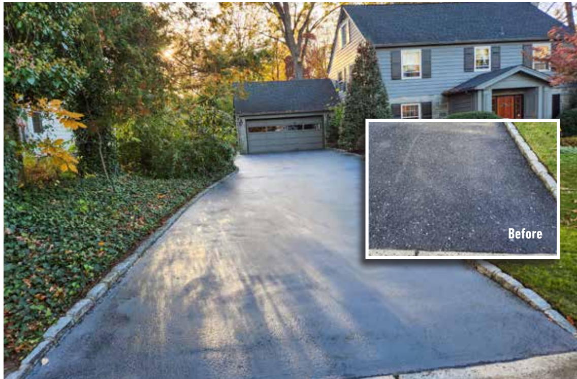
Powder pigment was added to the Surface Armor™ to achieve a similar finish to the original asphalt. The 1250 ft 2 driveway was completely resurfaced in approximately 5 hours.
