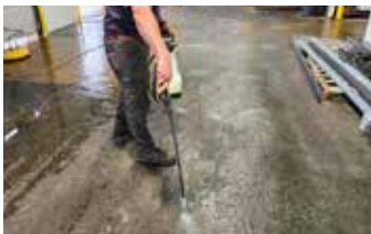
Clean floor with Pro-Grade Cleaner before applying Ecobeton® Vetrofluid.
