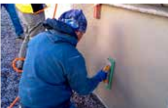
Using a grout float to apply the desired finish prior to the final application of Vetrofluid®.
