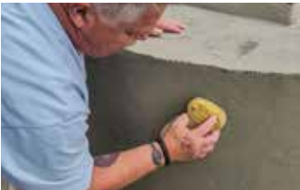
A damp sponge is used to smooth out the Surface Armor® and give it a soft texture.
