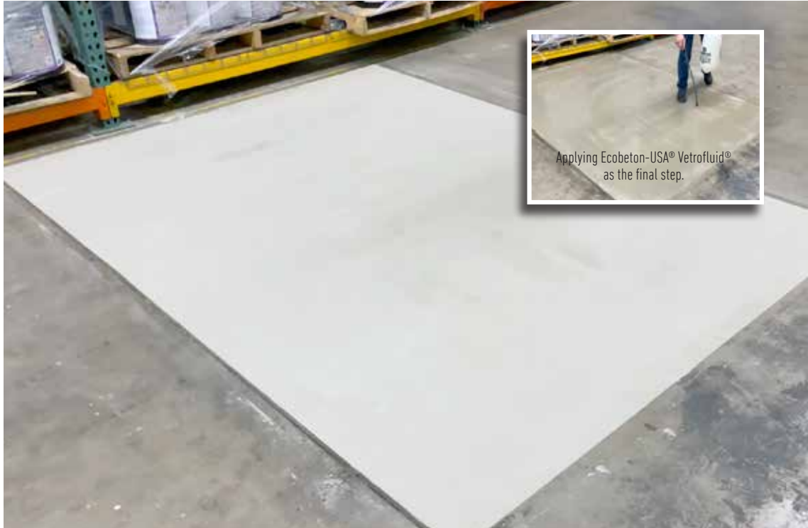
Warehouse floor panel brought back to 'new' appearance and ready for heavy forklift traffic. A light broom finish was applied to reduce a 'slip and fall' hazard.
