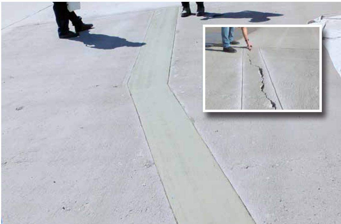
Filling cracks with Elephant Armor® using a roller and squeegee.
