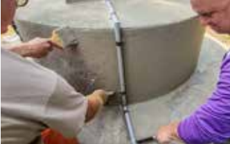
Apply Surface Armor® vertically using a brush, then use a Squeegee Trowel to remove brush marks.
