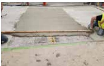
The center panel is filled with Elephant Armor® to the level of the two outside panels.
