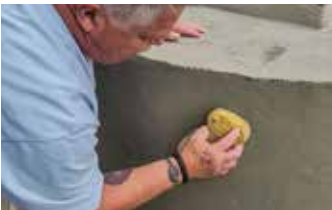
A damp sponge is used to smooth out the Surface Armor® and give it a soft texture.
