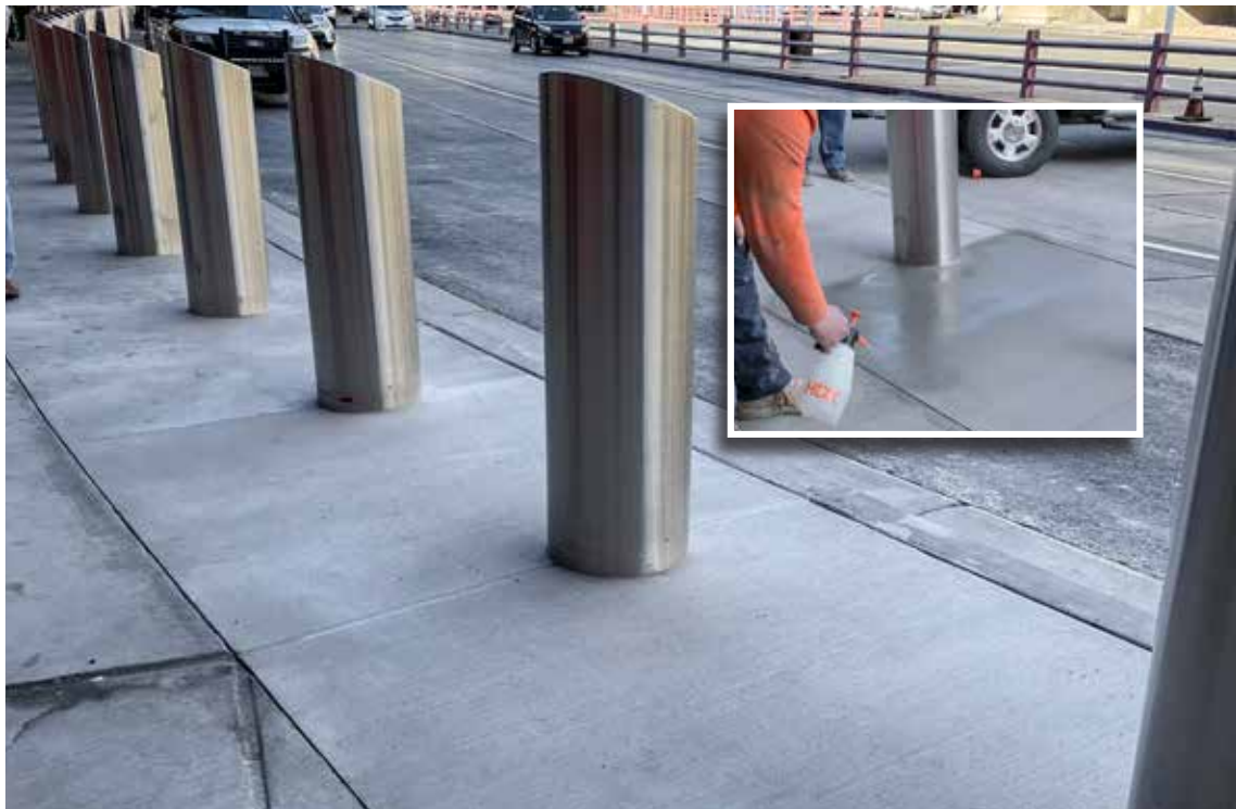
Finished panels showing a new appearance. Inset photo shows Ecobeton-USA Vetrofluid® being applied as the final step of the Surface Armor™ System.
