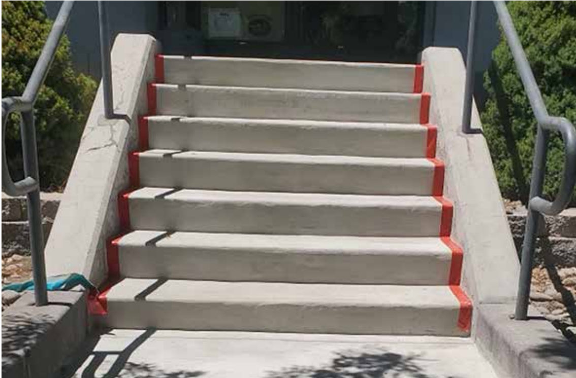
Severely weathered and broken stair treads made new, extending the lifecycle with Elephant Armor®. Repair completed by Morgan Construction, Reno, NV.
