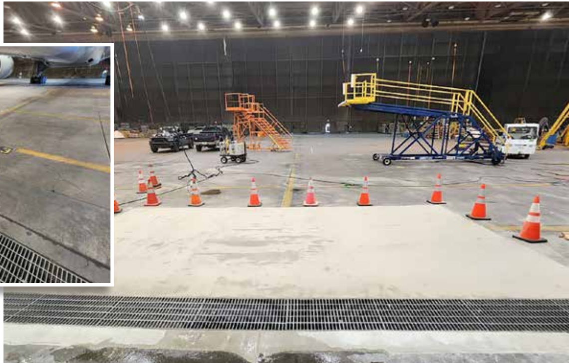
Photo showing extensive damage to the concrete around the drains, including a 3" 'point load' depression in the parking area at the jet's nose gear.
